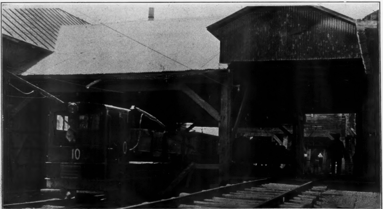
Train of Dump Cars Hauled by Electric Locomotive Dumping Mill Rock at the Primary Crushers
